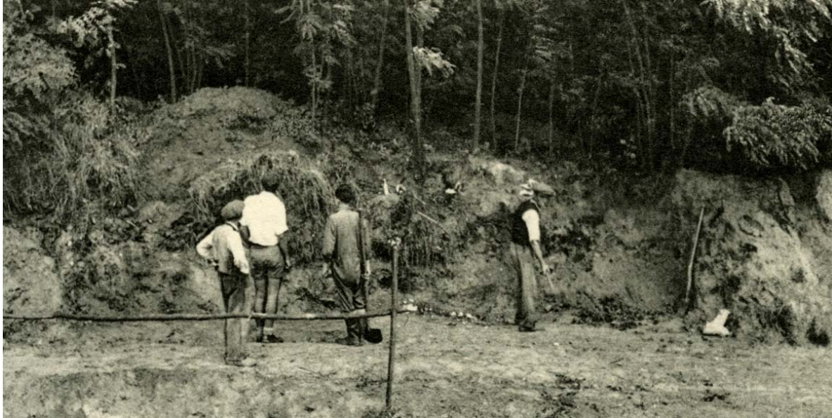
Figure 14. Beginning of the excavations of Glibert and Heinzelin in 1951.
